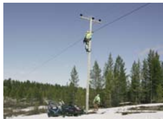
Because of frost, broadband cables are usually suspended from overhead electricity pylons rather than buried.
