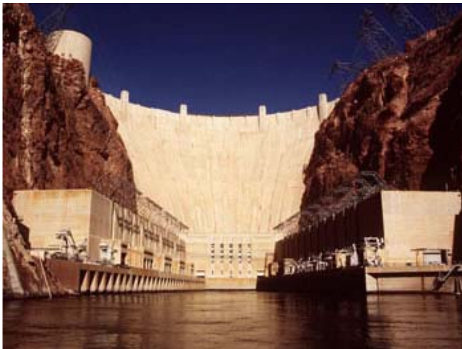
Conventional Hydropower – Hoover Dam
