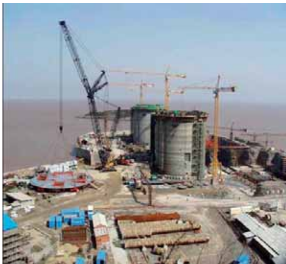
FIG. IV-1. Very heavy lift crane at Qinshan, China.
