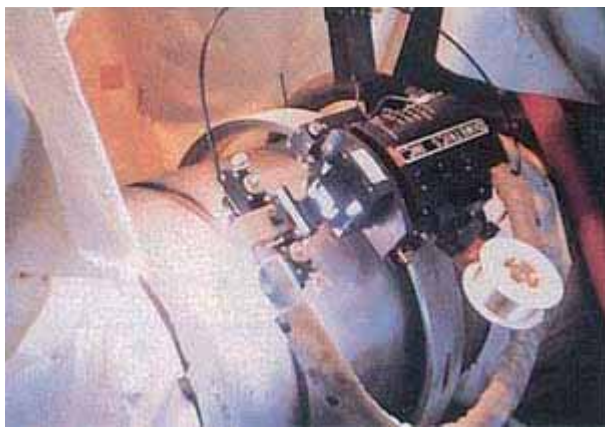
FIG. IV-10. Automatic piping welding at Kashiwazaki Kariwa-7 in Japan.
