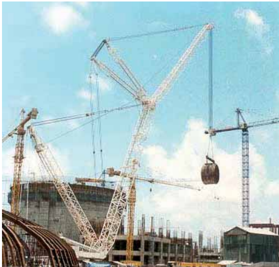
FIG. IV-6. Lifting the calandria at Tarapur-3 in India.
