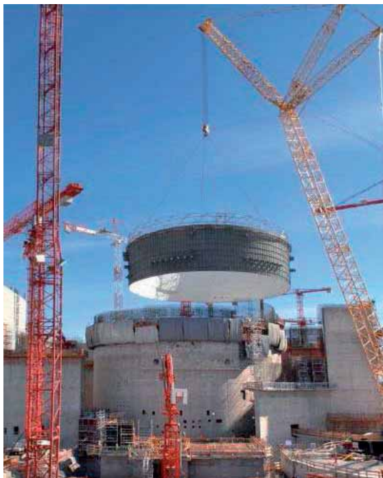
FIG. IV-3. Lifting the containment liner double rings at Olkiluoto-3 in Finland.
