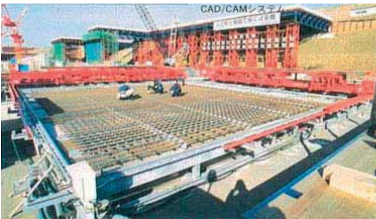
FIG. IV-13. An automatic rebar assembly machine at Kashiwazaki Kariwa-7 in Japan.
