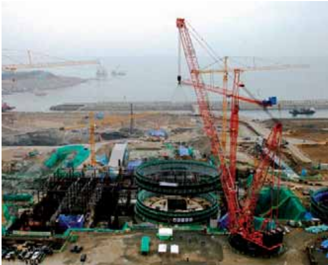
FIG. IV-9. Modularization of the containment liner plate assembly at Shin-Kori-1 in the Republic of Korea.
