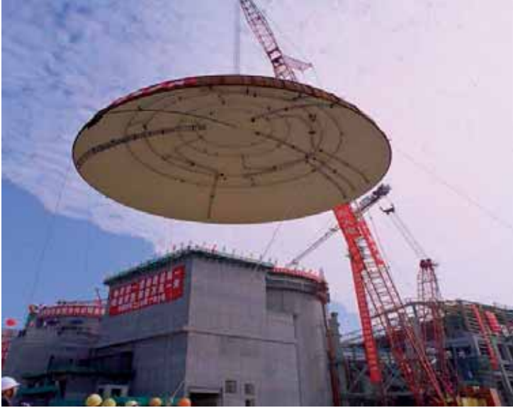
FIG. IV-8. Lifting the dome module into place at Lingao-4 in China.
