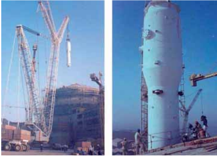
FIG. IV-5. (a) and (b): Installing a steam generator at Tarapur-3, India.
