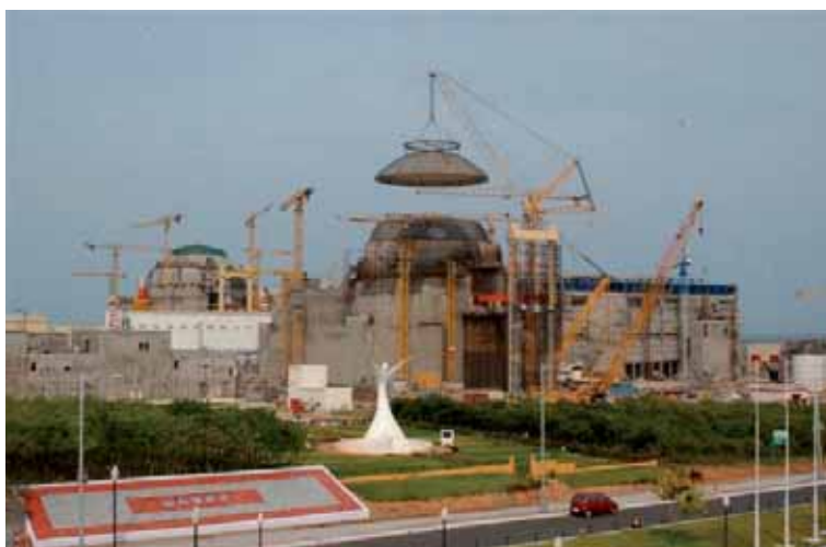
FIG. IV-4. Lifting the WVER-1000 containment dome into position at Kudankulam, India (photo credit: NPCIL).
