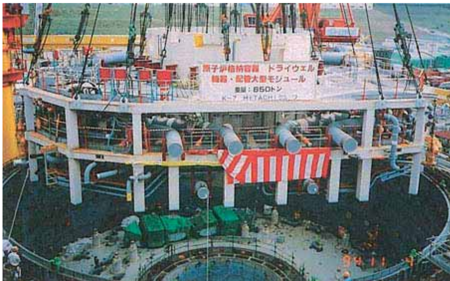
FIG. IV-7. Installing the upper drywell super large scale module at Kashiwazaki Kariwa-7 in Japan.
