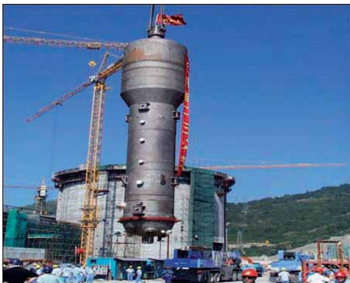
FIG. IV-2. Installing a steam generator at Qinshan 3-1 in China
