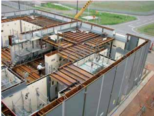
(b) Steel plate reinforced concrete.
